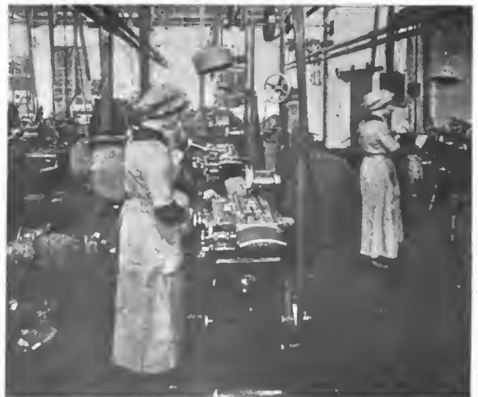
Performing surface grinding operation
